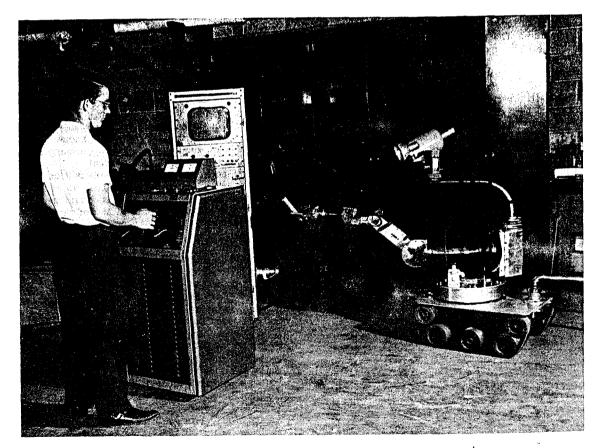
Fig.1 Remotely controlled mechanical robot used in plant recovery operation.
