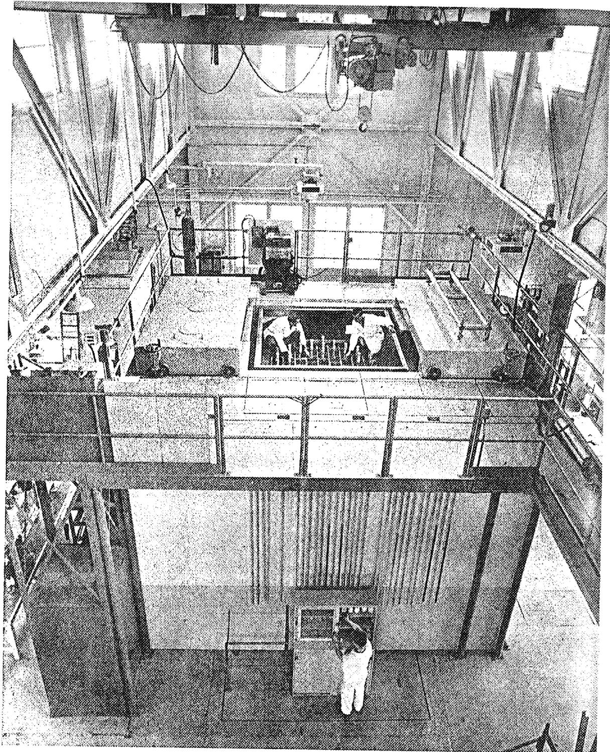
ZEEP (Zero Energy Experimental Pile), the first nuclear reactor outside the United States, was started up September 5, 1945, at Chalk River, Ontario. It was heavy-water-moderated and was used to assist in the design of the NRX. (Courtesy of AECL-Research)
