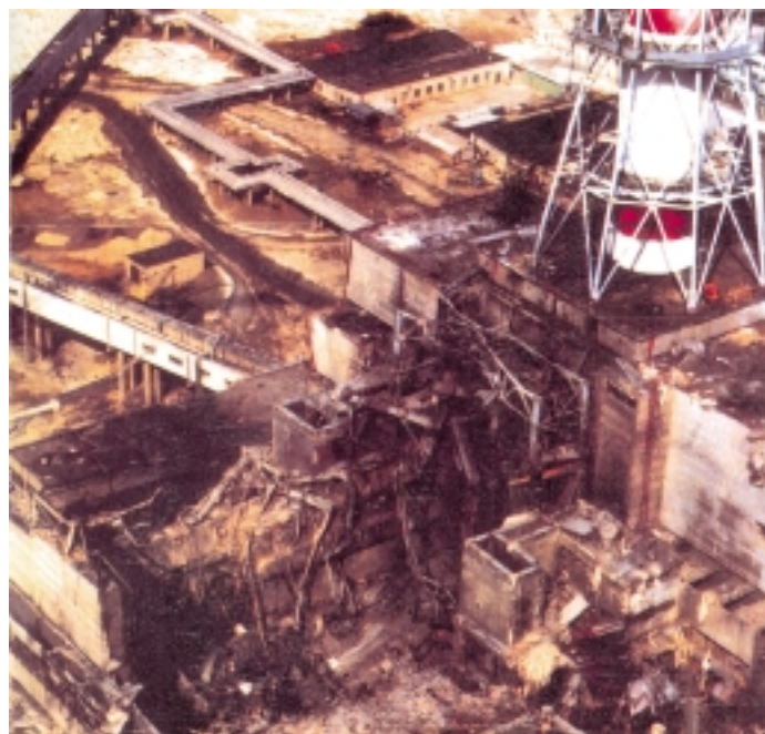
Unit 4 of the Chernobyl Nuclear Power Plant is shown several days after it suffered two explosions that destroyed the 200-tonne reactor core and the reactor building. Five to 10 tonnes of relatively heavy radioactive particles (predominantly strontium, plutonium, and other nonsoluble radionuclides) were blown out of the burning reactor and settled in the 30-kilometer exclusion zone around the plant. Smaller particles were carried great distances by a plume of smoke and debris ascending from the burning reactor.
