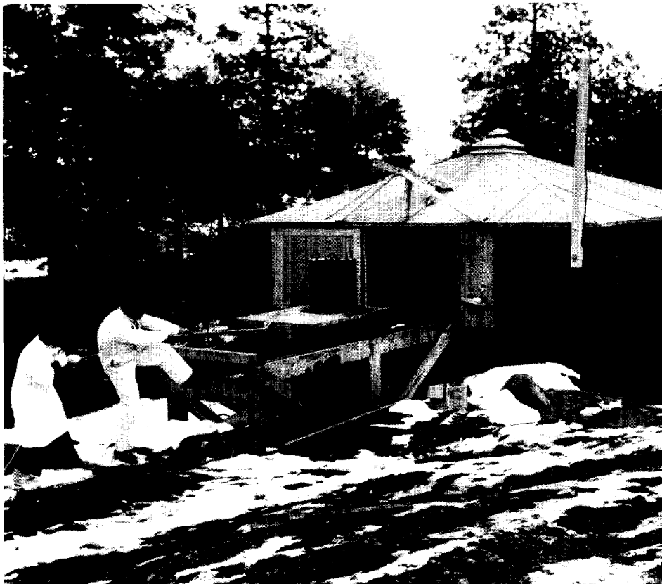
Wartime photo showing transfer of a heavily shielded gamma-ray source at the RaLa chemical processing site in Bayo Canyon. Motive power is being supplied by group leader Gerhart Friedlander and anchorperson Norma Gross, a WAC assigned to Los Alamos. Such sources were used to study the process of implosion, a method for achieving a critical configuration of the fissionable fuel in a nuclear weapon.
