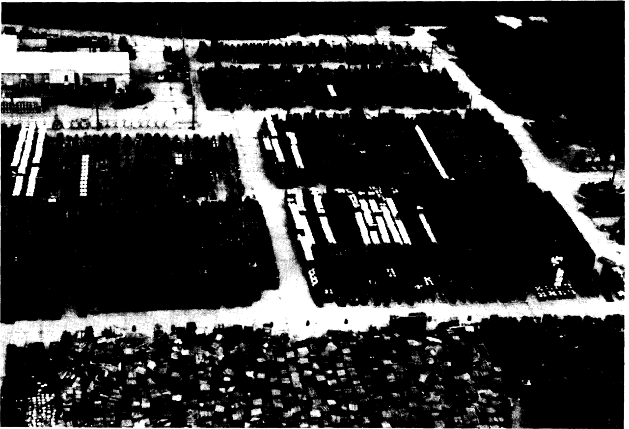
Photo credit: U.S. Department of Energy
