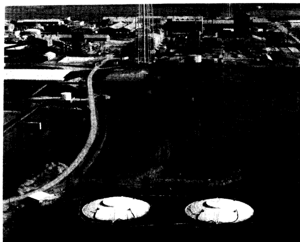
Photo credit: U.S. Department of Energy
