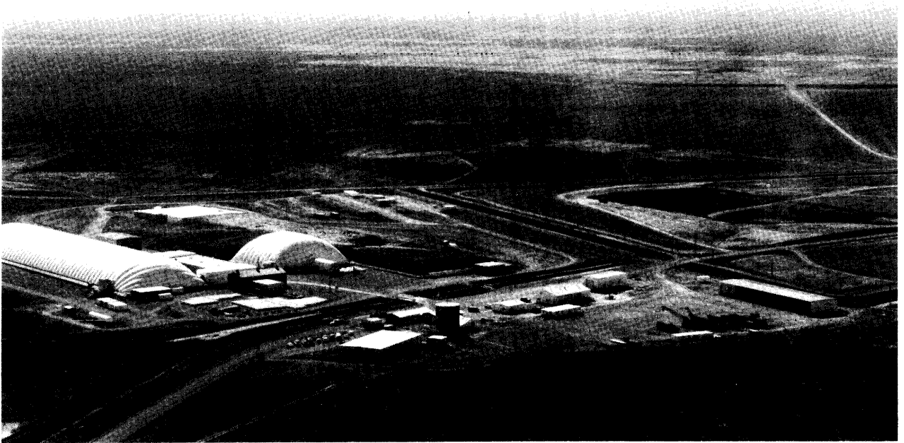
Photo credit: U.S. Department of Energy
