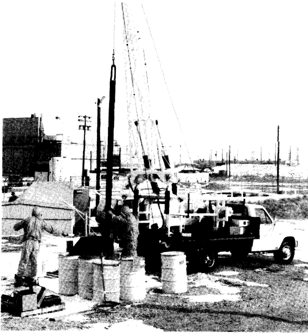
Photo credit: U.S. Department of Energy
