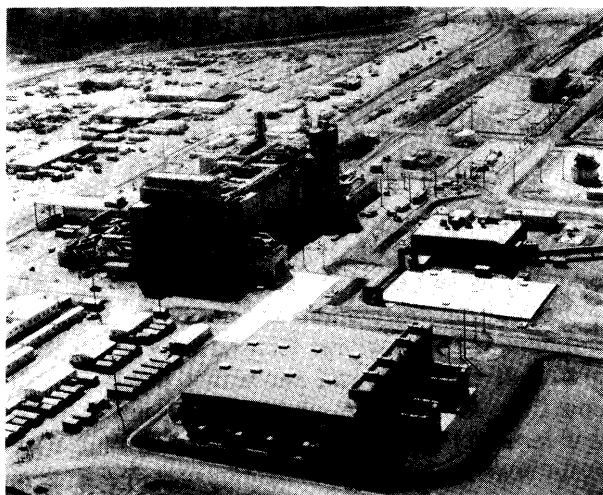
Photo credit: U.S. Department of Energy
