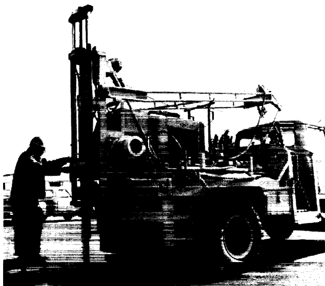
Fig. 17. Truck-mounted, auger-drill rig.
