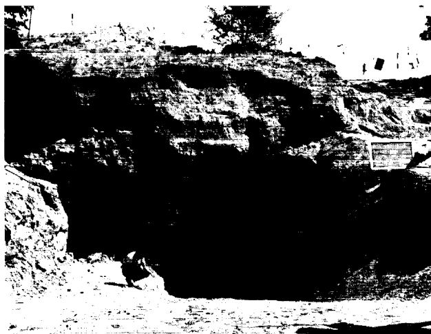
Fig. 83. Keyway excavation just north of H and Theta Buildings (looking north).
