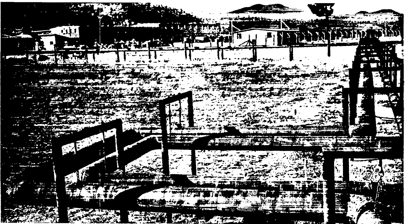
Fig. 34. Expansion loop in steam distribution line at S Site.
