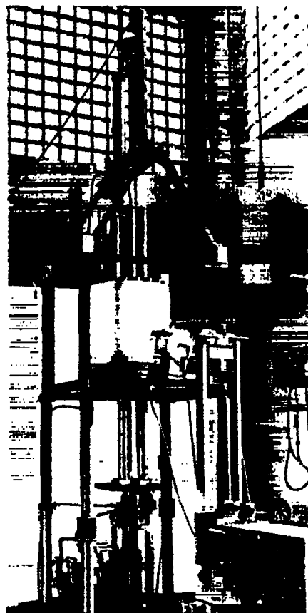
Fig. 21. The Aunt Polly mockup of the proposed Dumbo propulsion reactor.
